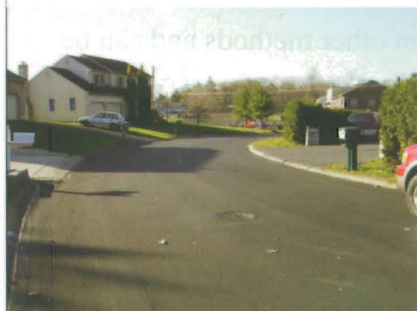
The final operation on Sunset drive was the application of a 3-inch hot mix super pave asphalt.
